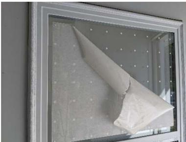
The tan pre-spacing/masking tape is engineered for easy release from the glass to leave the dots behind, but this adhesion to the dots need for the placement on the glass can become released with the rigors of shipping and storage.
